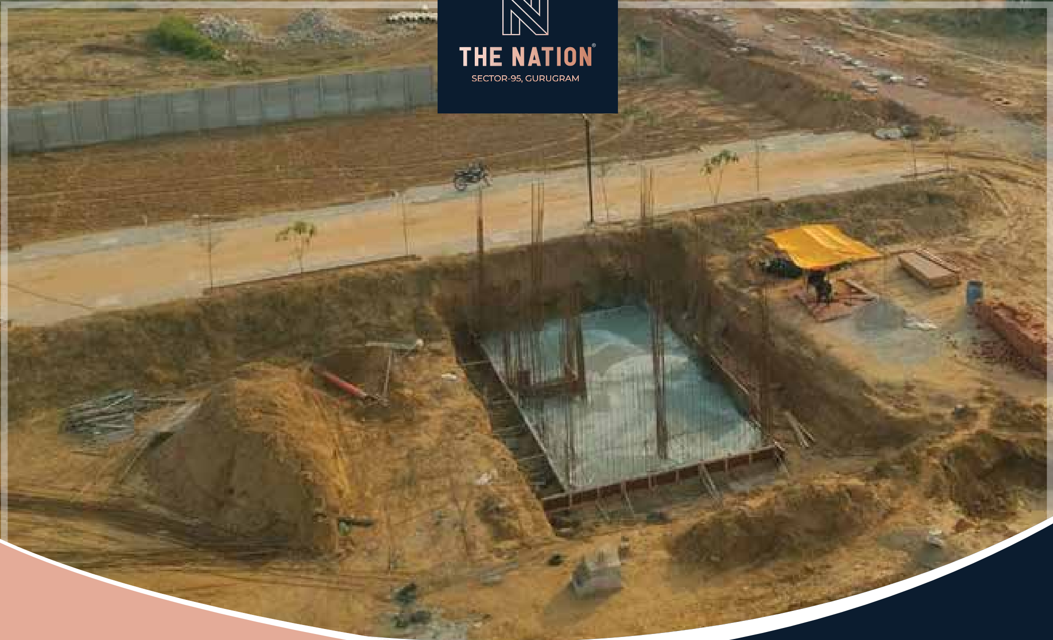
Floor Construction Work In Progress
